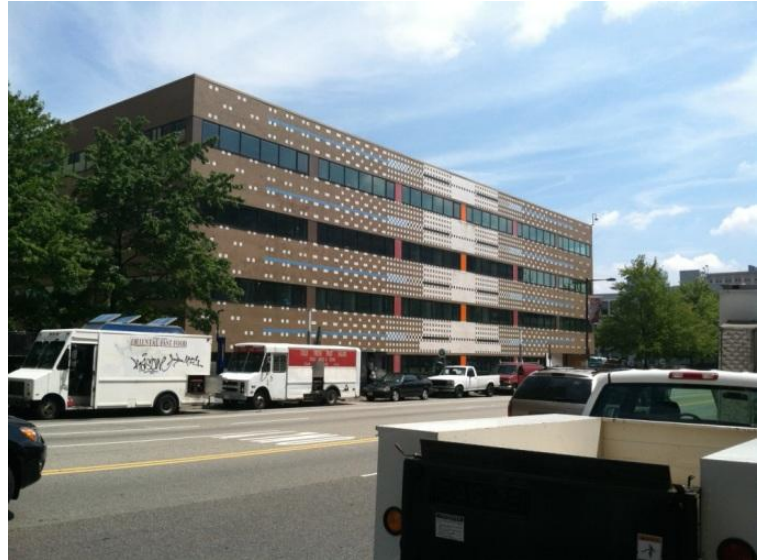
Figure 3: South Facade Of the URBN Center
